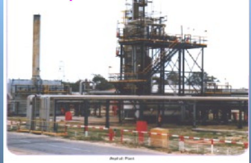
Azzawia Asphalt Plant
