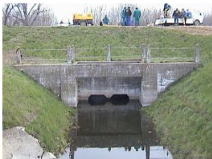
Figure 20. View of the Hatarmenti water-gate
