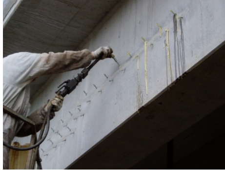
Figure 27. Reinforced PU grouting of the crack in the concrete construction
