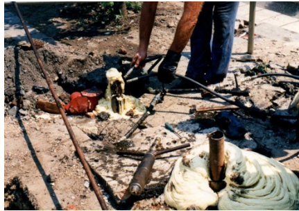
Figure 23. Sealing of the borehole with PU grouting
