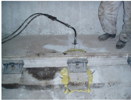
Figure 31. Detail of the grouting works
