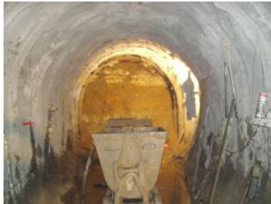
Figure 26. Grouted gravel in the face of the tunnel
