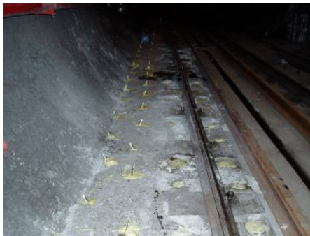
Figure 32. View of the railway after repair works
