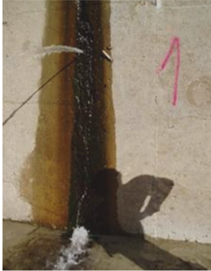
Figure 29. Dilatation joint before the grouting
