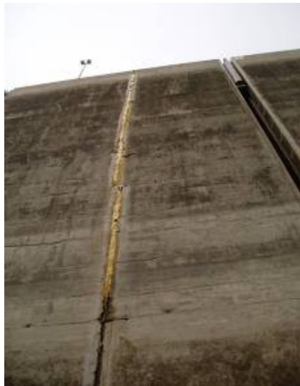
Figure 30. Dilatation joint after the grouting
