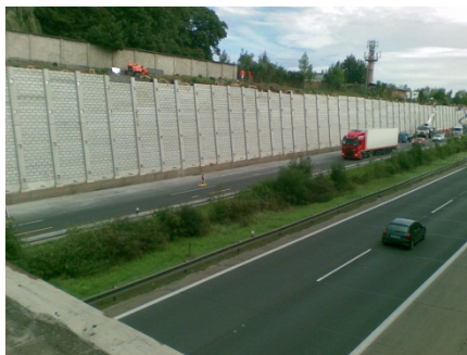
Figure 18. Situation before final completion of the works
